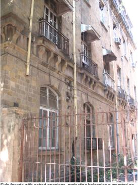
Side façade with ached openings, projecting balconies supported on brackets, sloping chajjas, modified openings to take in services
