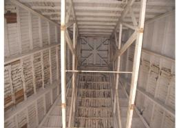
Wooden high sloping roof supported on wooden truss
