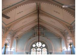
Ceiling with cross braced wooden sloping roof
