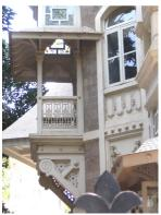
Wooden bracket detail supporting the projecting balcony
