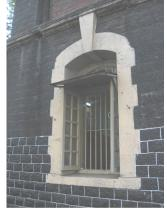
Grey stone clad façade with arched window with modifications made to the shutters and chajja
