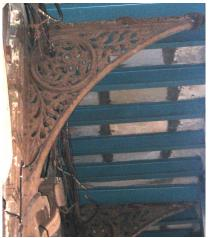
Cast iron bracket detail supporting the projection
